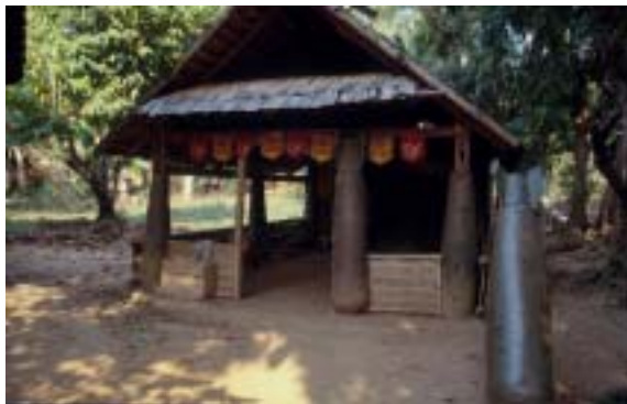
A house built of bomb shells as stilts in Muang Ngoy.
